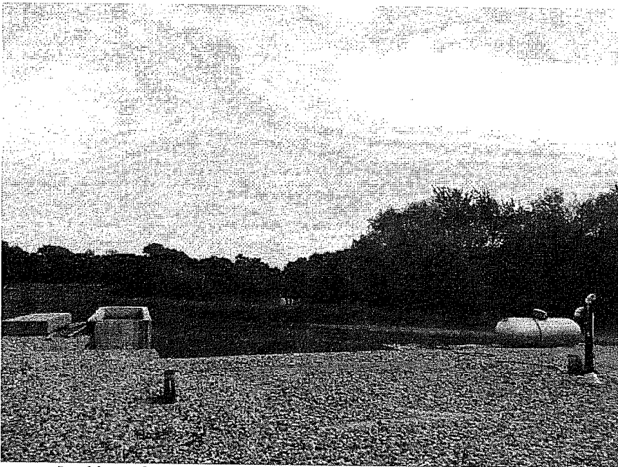
Looking E from the Unused Foundation and Basement on East Parcel
